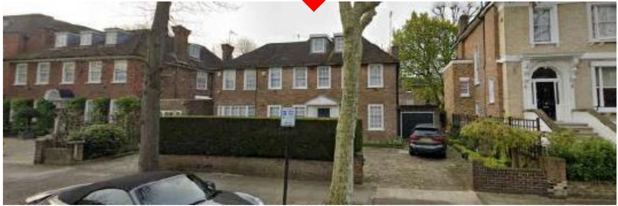
Front Elevation (No 47 Springfield Road to the left and No 41 Springfield Road to the right)
